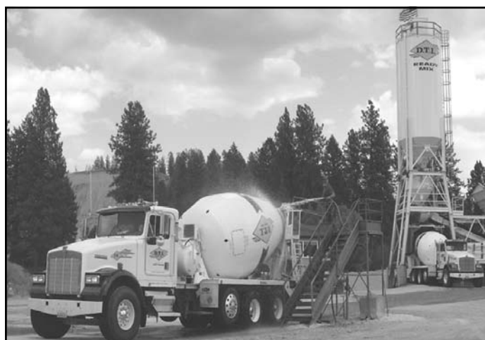
One D.T.I. Ready Mix truck gets a washdown (foreground) while another loads up with concrete (background). Photo Huckleberry Press.
